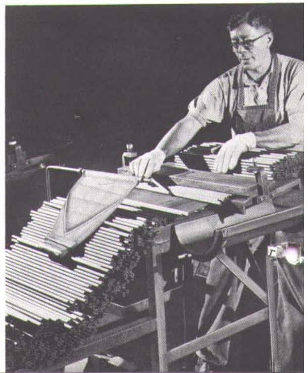
7. Straightness test is vital
