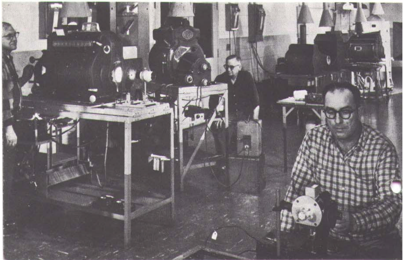
11. "Burn room" for testing performance
