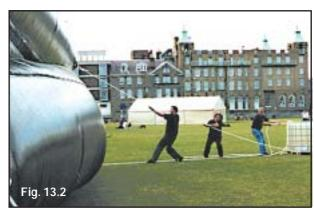
Release the guy rope gradually keeping tension on the rope at all times. Check that the fold is always in the middle.
