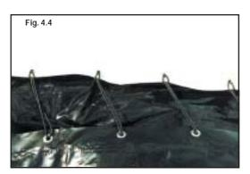
In the corners, do not necessarily match up the eyelets; just ensure that the screen is square in the space, see figure 5.
