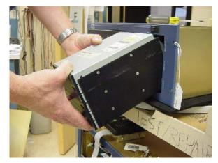
Figure 11. Loosen screw and remove drives
