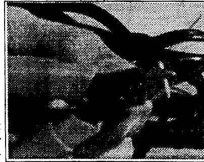
Make sure the stranded shield wires are twisted together and no stray strands touch the inner conductor that can cause a short circuit.
