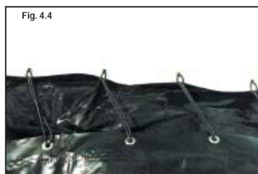
In the corners, do not necessarily match up the eyelets; just ensure that the screen is square in the space, see figure 5.
