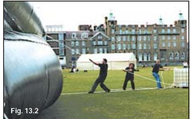
Release the guy rope gradually keeping tension on the rope at all times. Check that the fold is always in the middle. The frame will gradually rise. The people securing the frame from the back must not let too much rope out. Both front and back ropes must be counterbalancing. The aim is to keep the top of the frame as near vertical over the bottom as possible during inflation.
