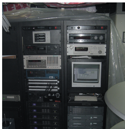
▲ The Planetarium's surround sound system consists of two Peavey Cinema Acoustics CAS 3118 subwoofers and six Peavey Cinema Acoustic CAS 5115 loudspeakers, driven by seven QSC Audio DCA-1622 power amplifiers.
