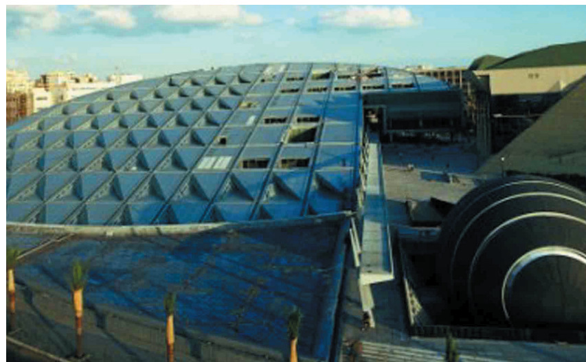
▲ Spitz of Chadds Ford, PA designed and installed the Bibliotheca Alexandrina planetarium (pictured in the lower right corner) video system, and the planetarium's audio system was designed and installed by MegaSystems of Wayne, PA.
